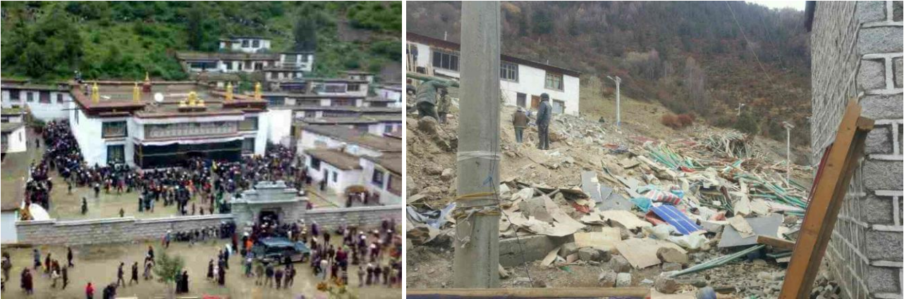
Images of Jhada Gon Palden Khachoe before and during the demolition
